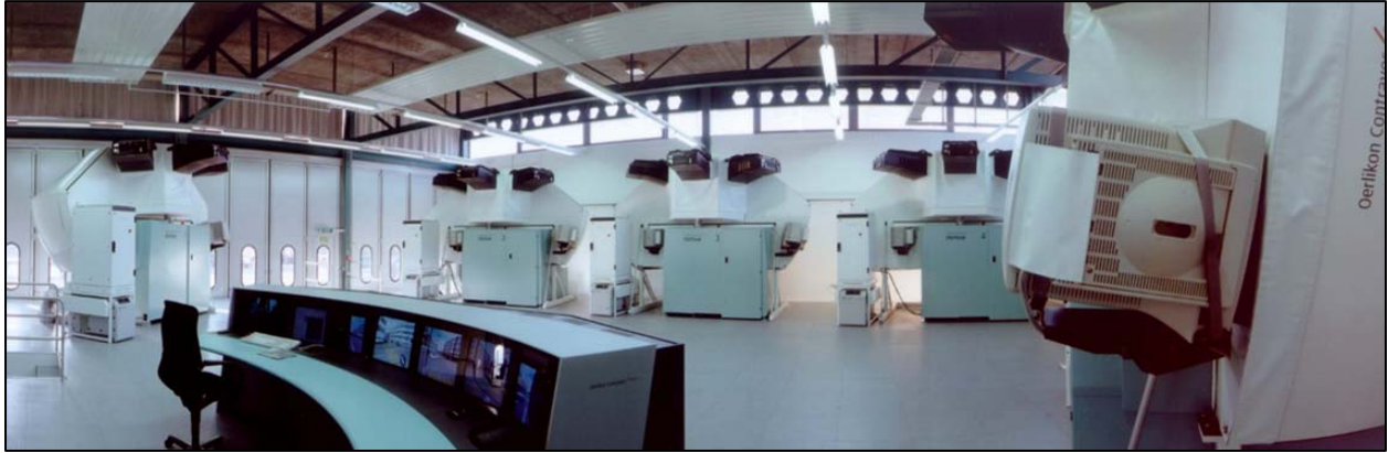
Target simulator bank installed at customer's site
