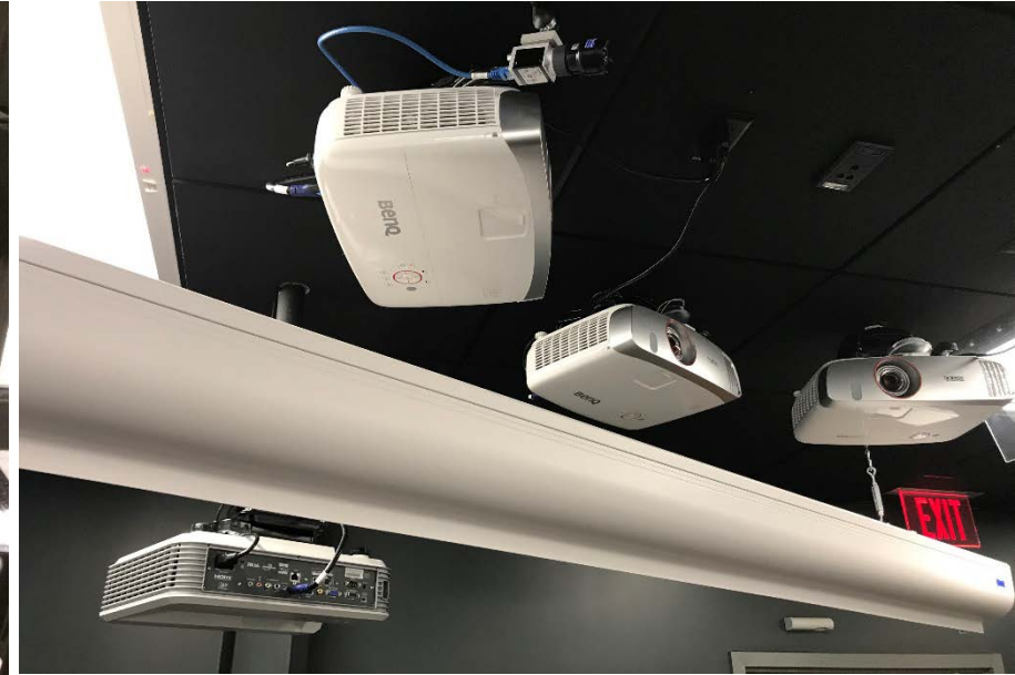
Clean Projector and Alignment Camera Installation
