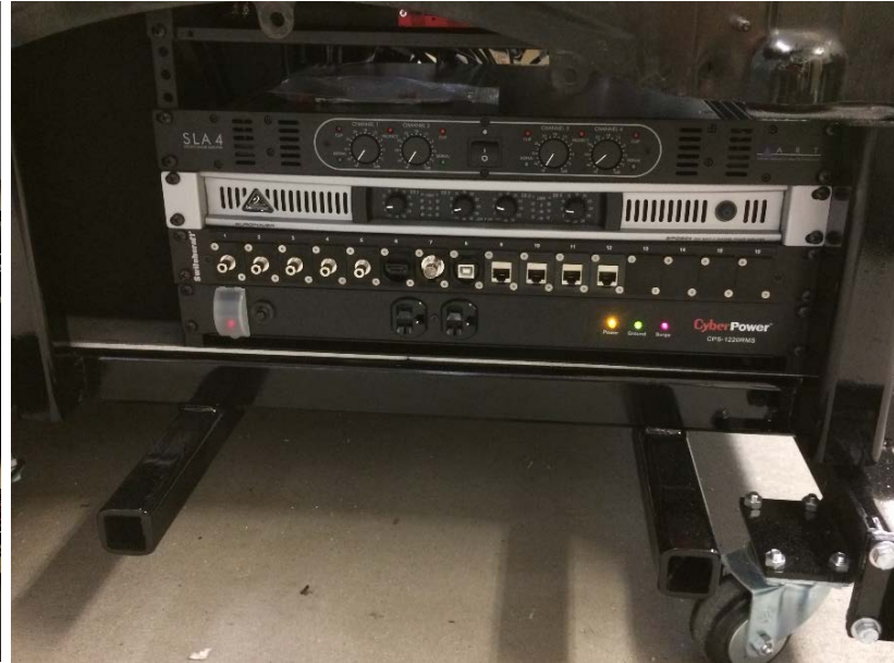
All Connections in Passenger Wheel Well
